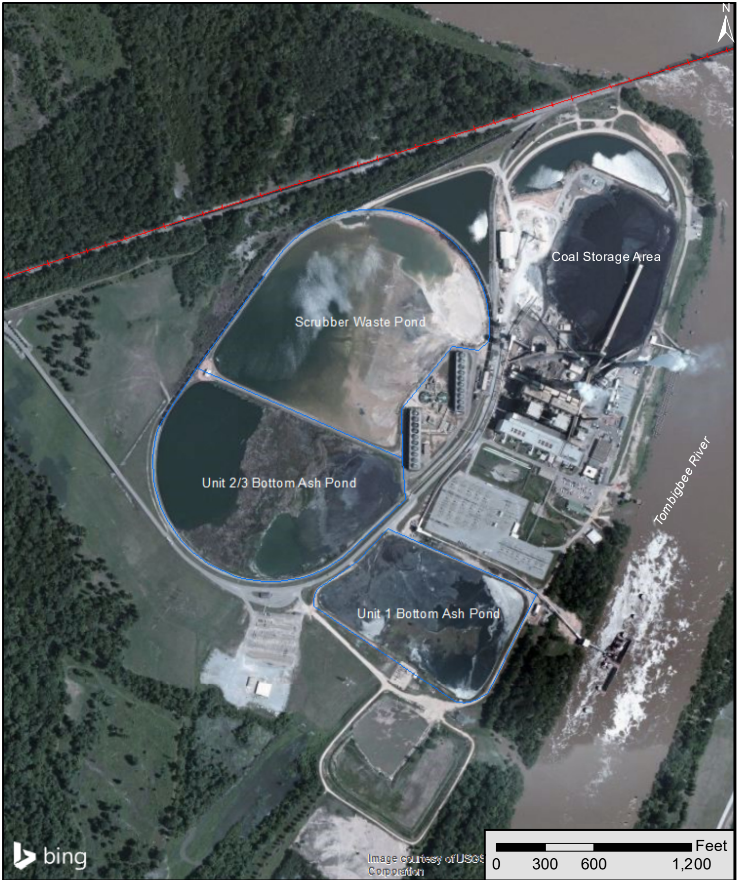
Figure 2 - Aerial Map of Impoundments Charles R. Lowman Power Plant PowerSouth Energy Cooperative Leroy, AL
